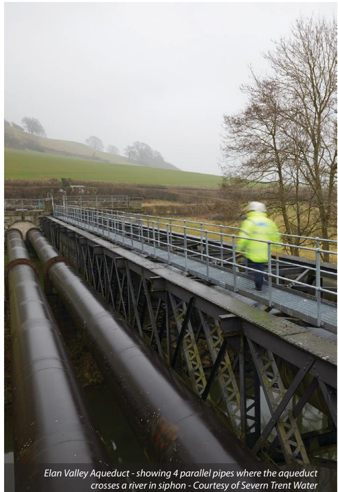
Elan Valley Aqueduct - showing 4 parallel pipes where the aqueduct crosses a river in siphon - Courtesy of Severn Trent Water
