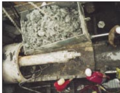
Photograph above. Mucking out to enable the TBM launch
