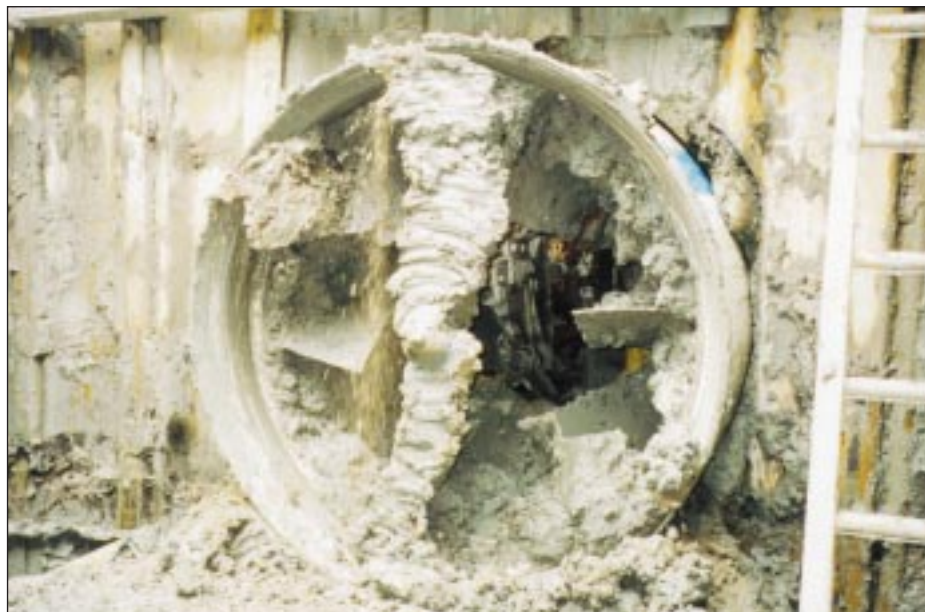
Photograph Above. TBM breakthrough
