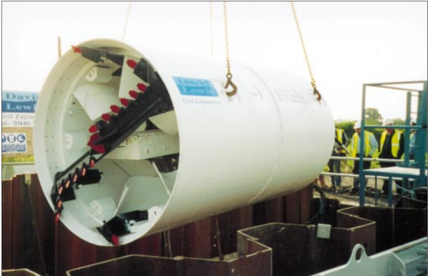
Photograph Above. The first launch of the brand new Akkerman 1500 TBM
