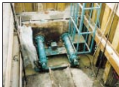
Photograph Above. The jacking set up in the drive pit
