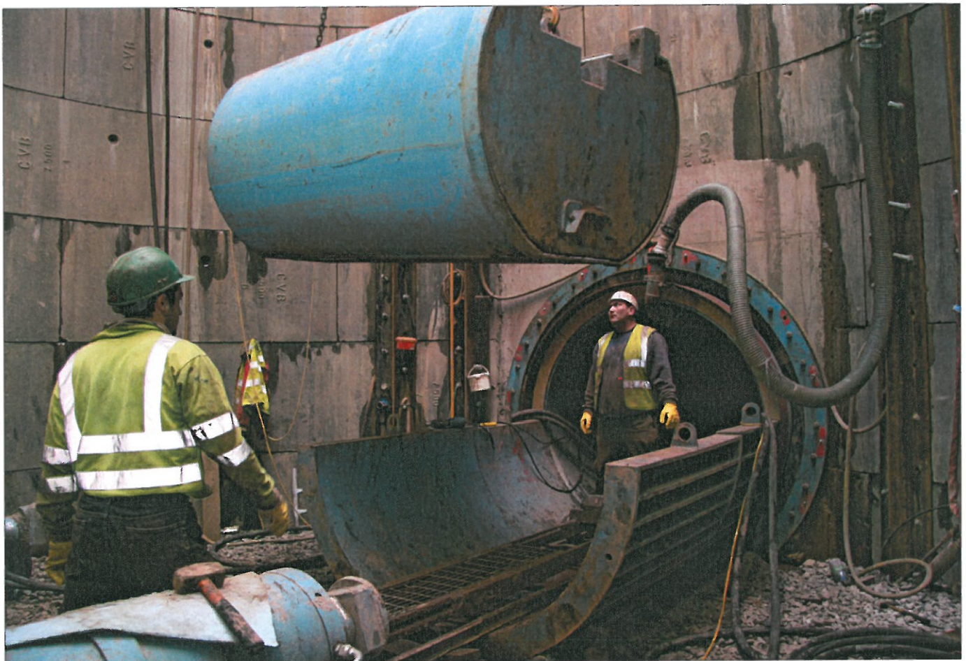
Photograph Above. Mucking out on the Akkerman drive. (Library)
