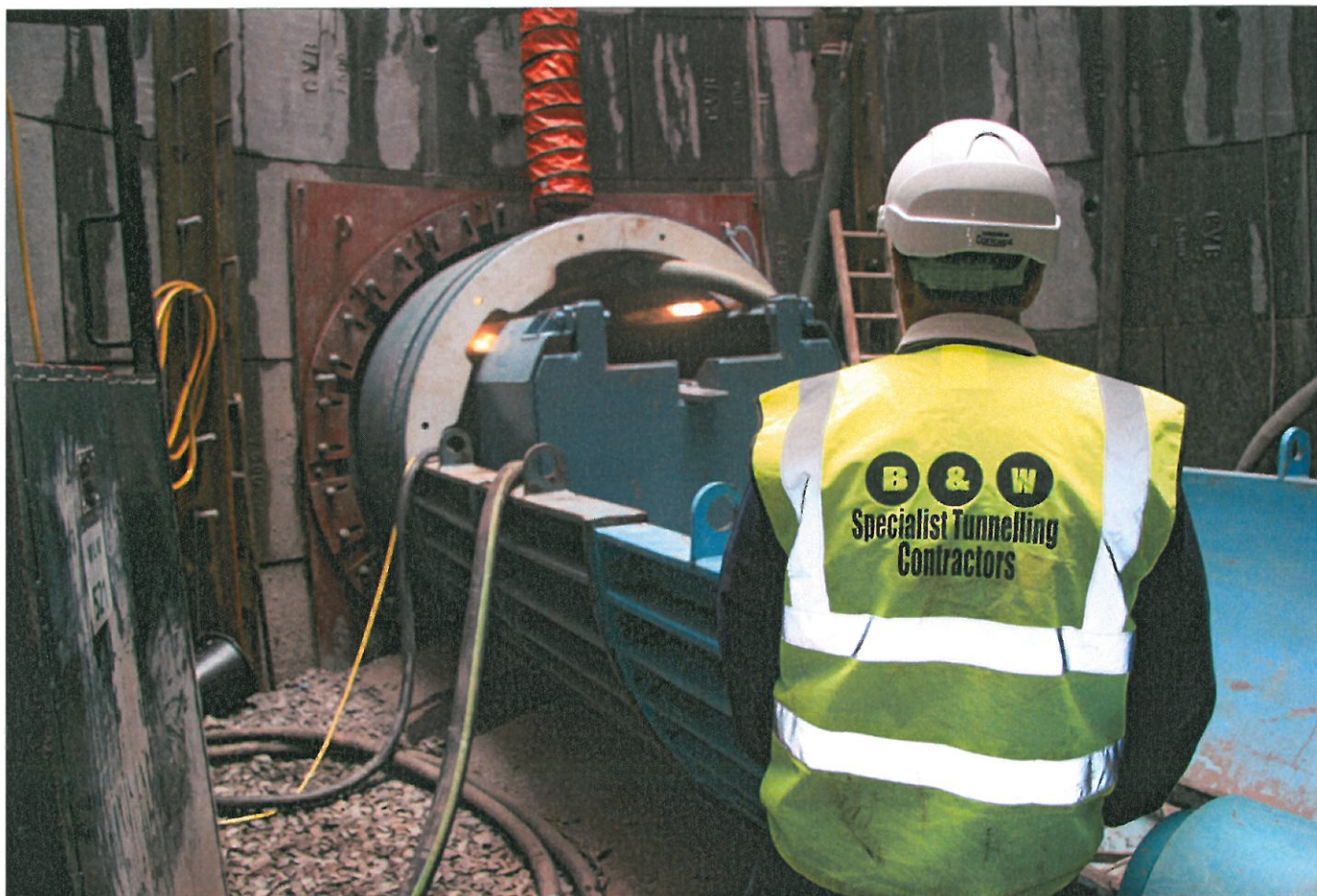
Photograph Above. The TES 1800 EPB TBM mucking out the sandstone (Library)
